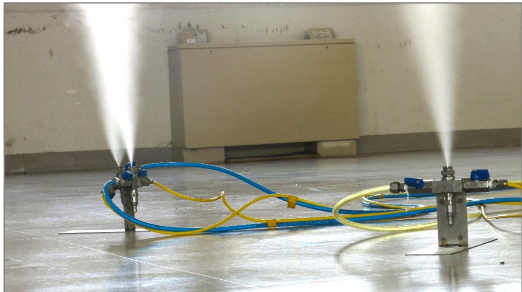
Figure 15. Dry-fog being applied via spray nozzles in Building 6733.
