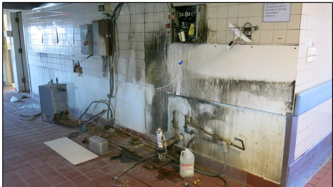
Figure 4. Kitchen area inside Building 2261
