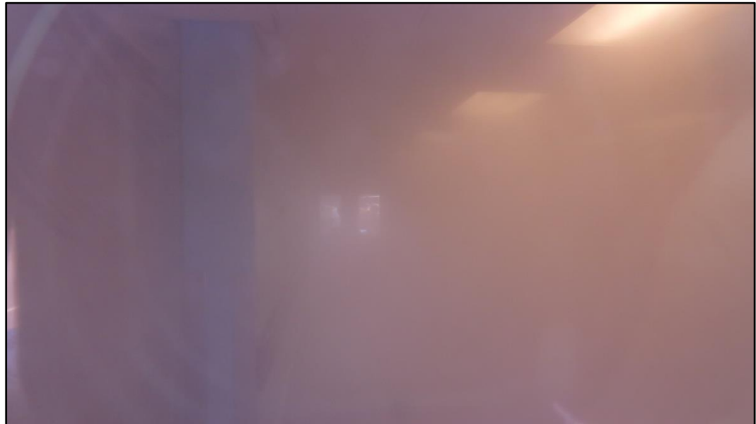
Figure 17. Dry-fog accumulation in kitchen area within Building 2261.
