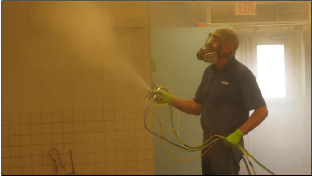
Figure 14. Dry-fog being applied to intake of HVAC ducting Building 2261.
