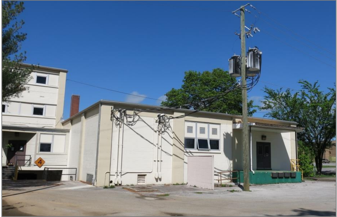
Figure 6. Exterior of Building 6733 – barracks
